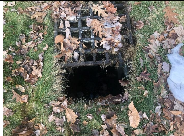
Photo 2: New 4-way shallow catch basin
