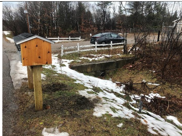
Photo 1: 3 Culvert under entrance to storage facility
