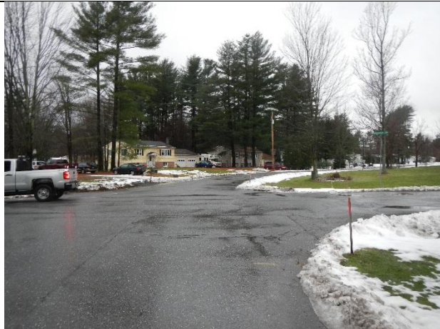
Photo 1: 3 dry wells at Hemlock/Woodcrest
