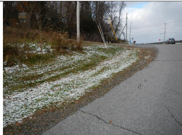
Photo 2: Grassed ditch along Howard Drive
