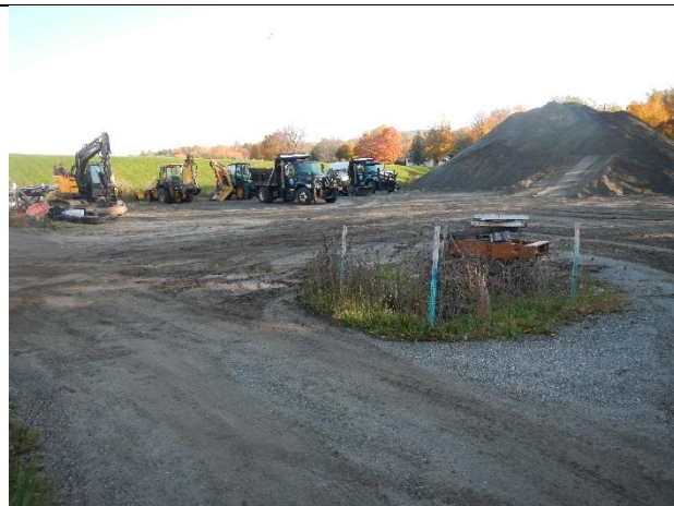
Photo 1: Large gravel/dirt area draining to catch basin
