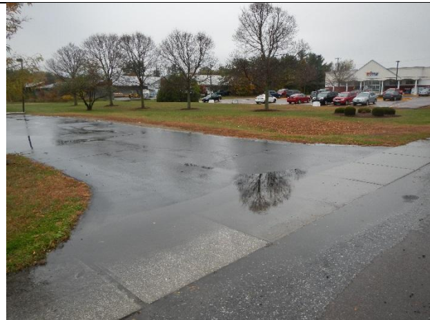
Photo 2: Fabric filter installed under catch basin grate
