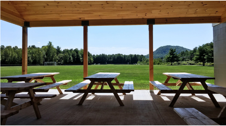
Bombardier Park Fieldhouse Pavilion
