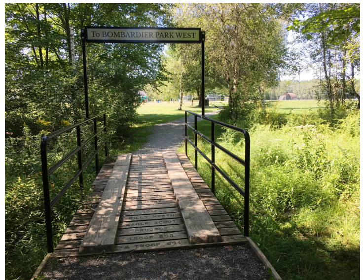
Bridge to Bombardier Park West
