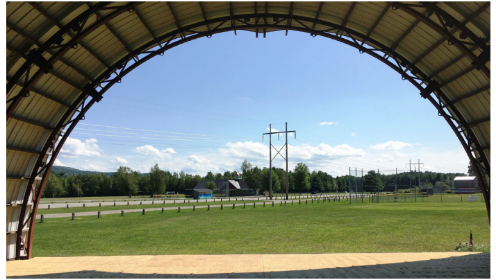
Milton Outdoor Performance Center
