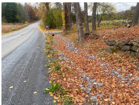
Figure 4. Beebe Hill Road (South) Stone-Lined Ditch.
