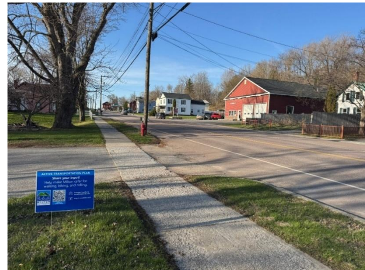
Photo 1. Sidewalk on the western side of River Street in Milton.
