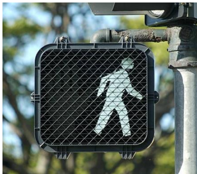
Photo 32: Pedestrian Signal (Source: FHWA)
