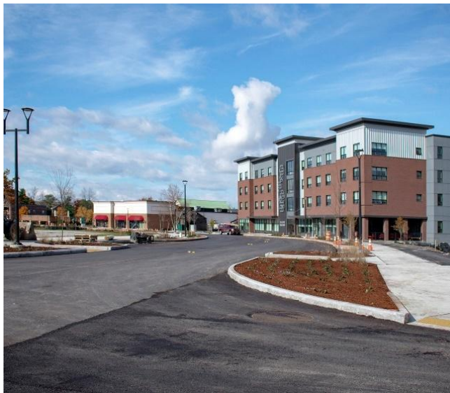
Photo 30: Curb Extension along Market Street (Source: City of South Burlington)
