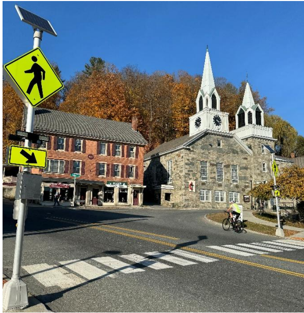
Photo 31: Existing RRFB on Main Street (VT 11) in Springfield, VT (Source: VHB)
